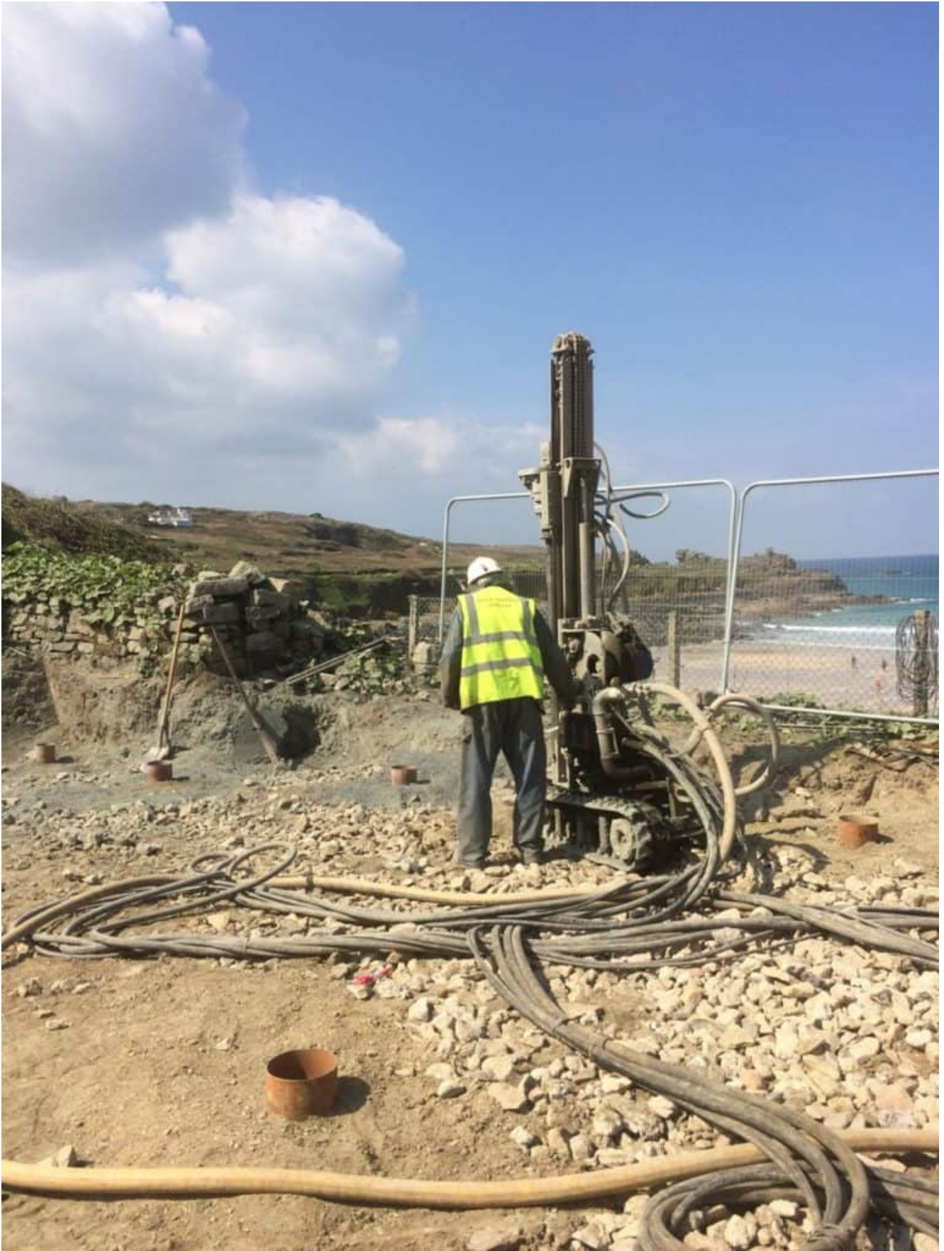
Aquasource SW Ltd has been piling at Porthmear Beach, St Ives for a new build house.
