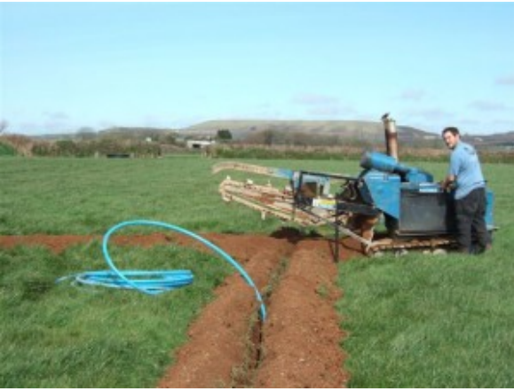
Pipe Laying with Chain Trencher
