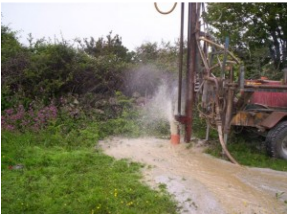
Drilling for Water, Just Starting to get wet!
