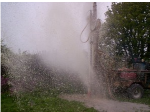
Drilling for Water, plenty
