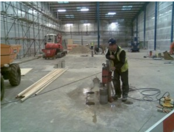
Concrete Core Drilling
