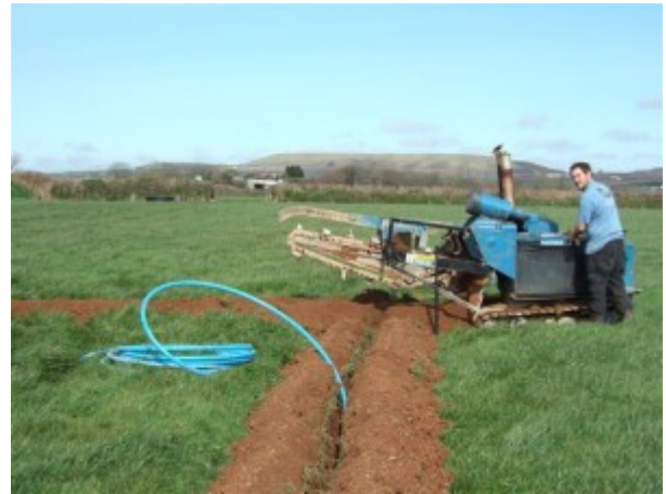
Pipe Laying with Chain Trencher
