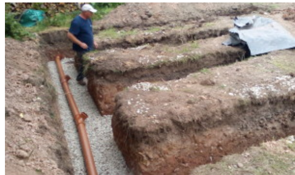
Drainage Field Excavated
