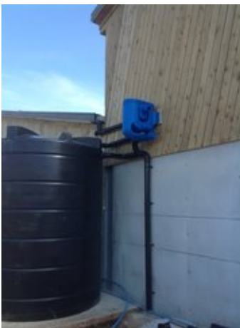
Rain Water Harvesting System on a Barn in Devon
