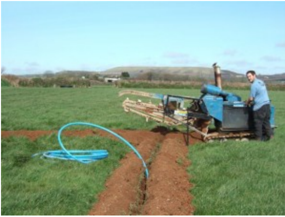
Pipe Laying with Chain Trencher
