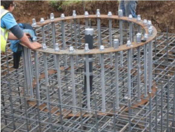
Wind Turbine Base Steel
