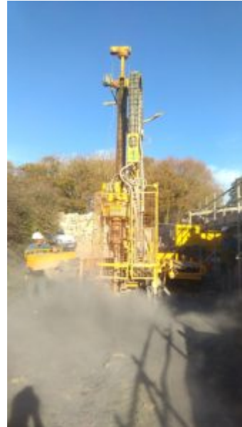
Groundsource Drilling in Cornwall
