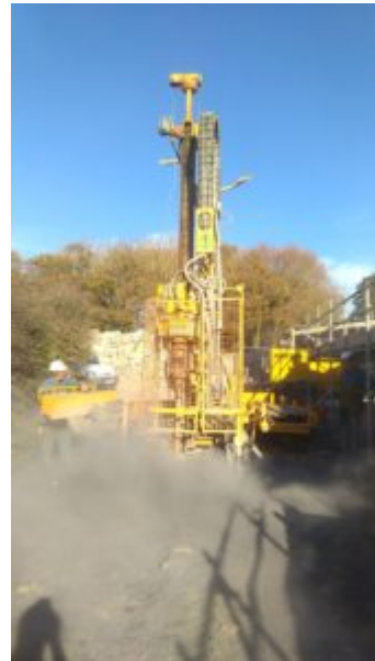
Groundsource Drilling in Cornwall
