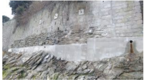
View of Sea Wall Repair
