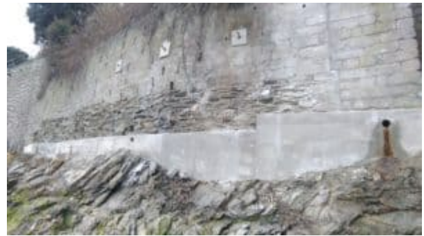
View of Sea Wall Repair
