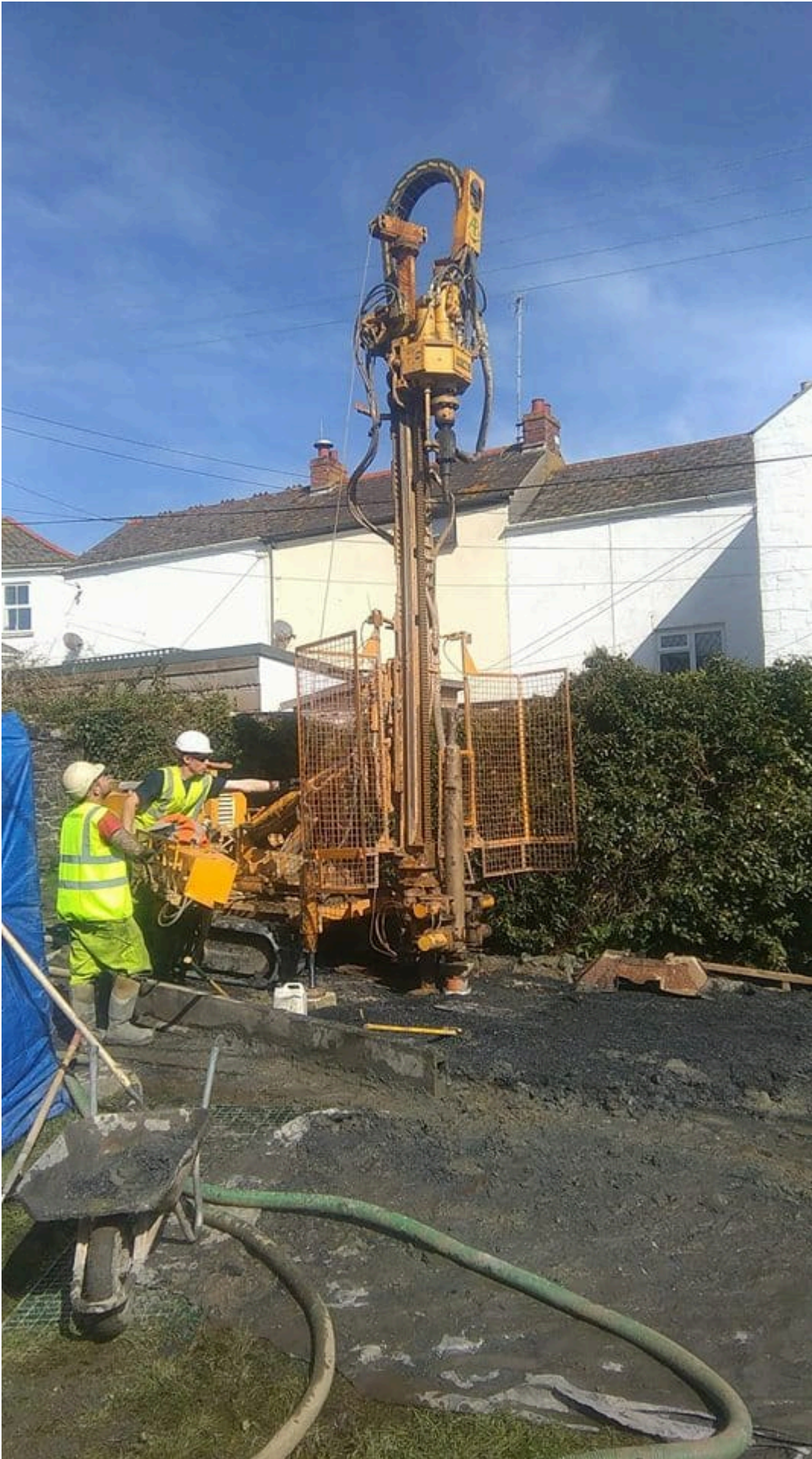
Drilling Ground Source Heat Pump Boreholes
